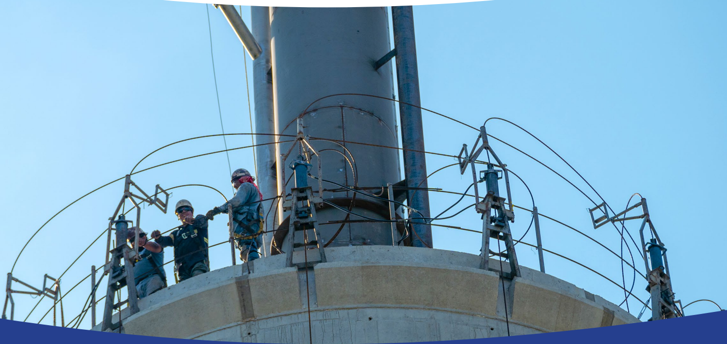
TWC's Alnwick water storage tank under construction.
