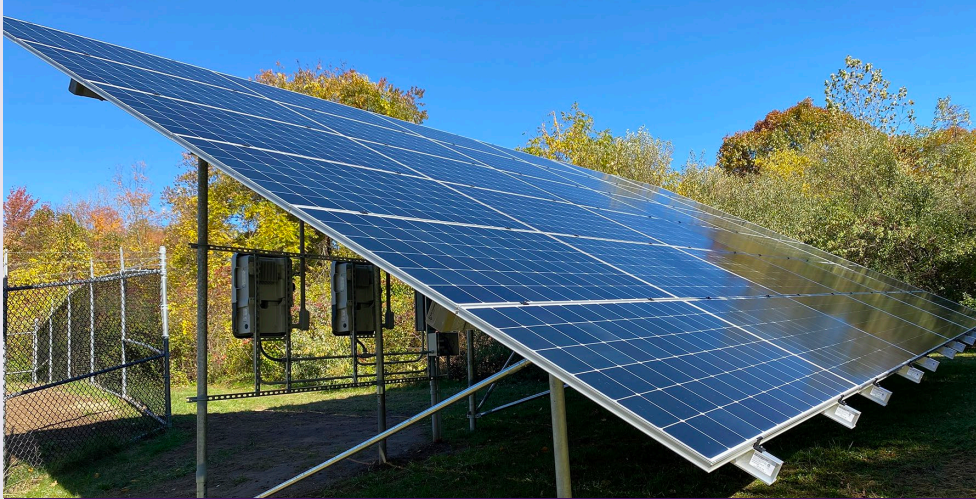
Colchester, CT — Connecticut Water completed the installation of solar panels at one of its smaller water systems that were sufficiently sized to fully meet energy requirements to pump, treat, and move water through the water system, effectively removing it from the power grid.
