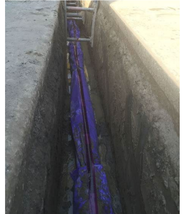
Purple recycled water pipe installation
