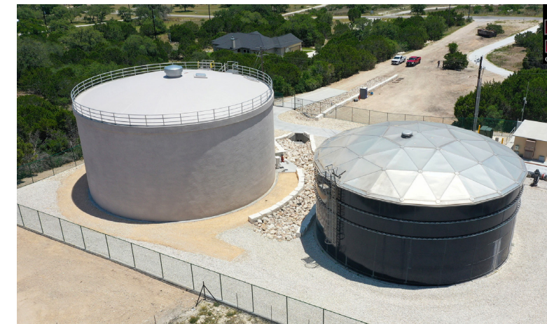
Comal County, TX – This 750,000-gallon water storage tank was completed at a cost of $2.2 million. It is one of 13 water storage projects completed, under construction, or in design.
