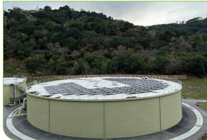
This solar-generation project atop the storage tank at our Belgatos station is capable of producing 140 megawatt hours of electricity each year.
