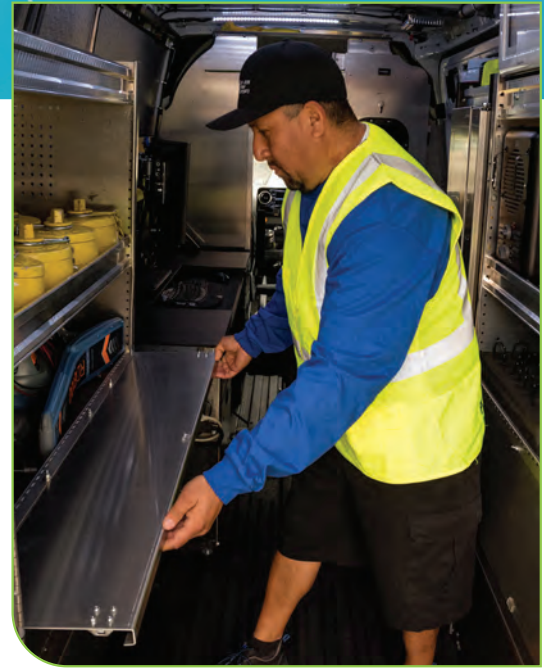
Hydrant caps with acoustic leak sensors loaded and ready for deployment in San Jose Water's distribution system.
